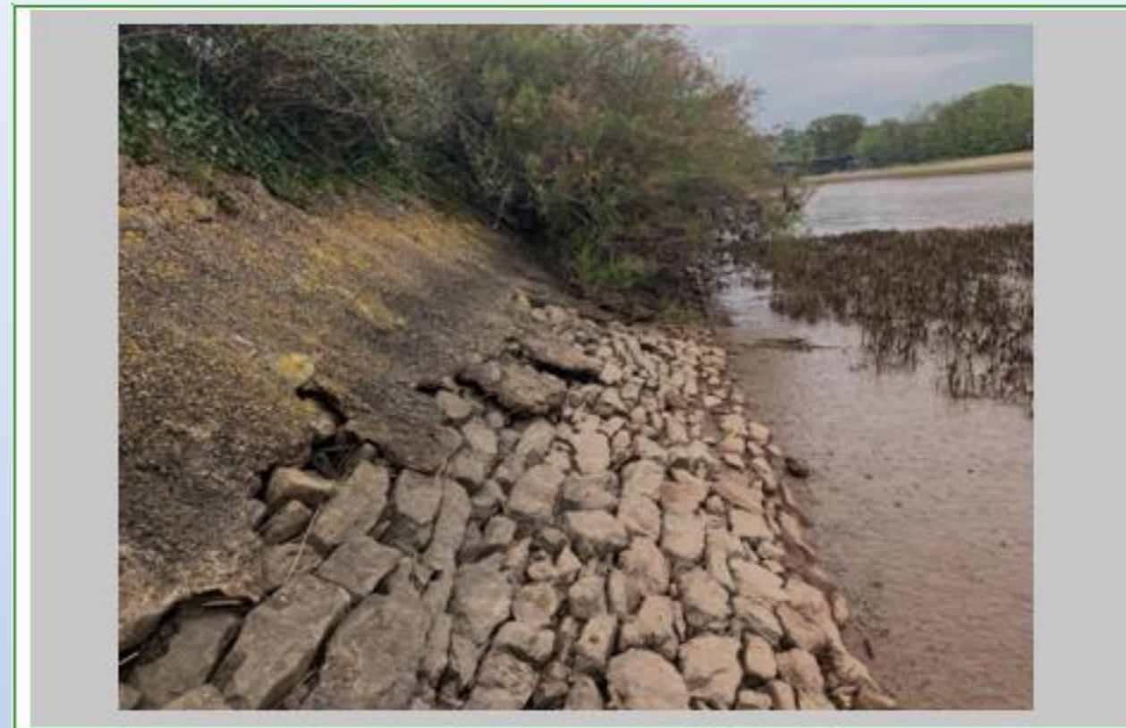
Figure 3: Photo of typical flood bank condition
